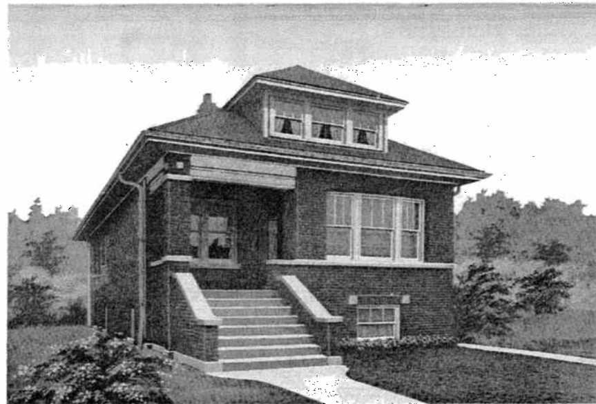
Many aspects of the design of the ubiquitous "Chicago bungalow" are Wright influences: overhanging hipped roofs, crisp lines, and art glass windows. Above, a design by the Radford Company, one of the largest suppliers of stock designs in the 1920s.
